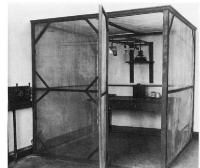
Figure 4: "Shielded cage room developed by the [National Bureau of Statistics] Radio Section in late 1917. This 'Faraday Cage,' as it was called, reduced the very strong signals from across the Potomac river from the Navy's strong signals broadcast at Arlington." Photo: NBS/NIST
